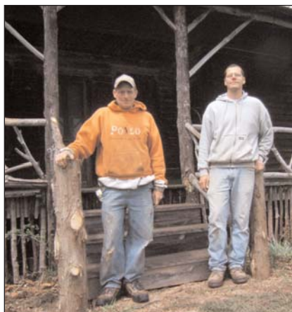
Timothy Bowen and Stephen Banks, members of the crew of Frank Furlan and Sons, pose at the porch in April after installing sturdy cedar posts.
